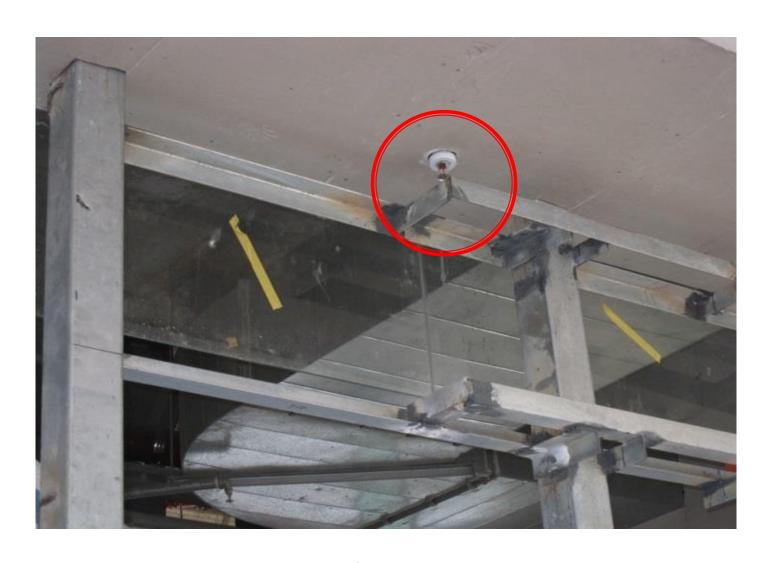
**x** Blockage of sprinkler head
