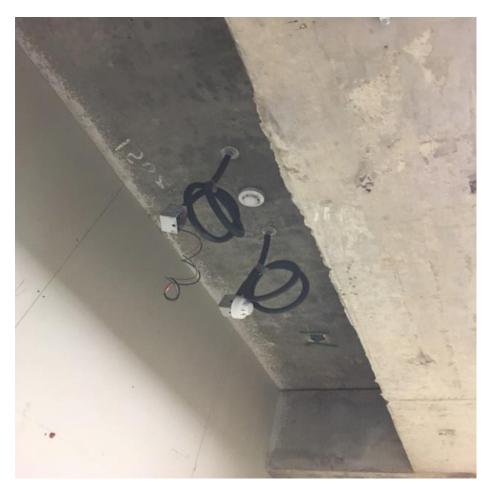
**x** Incomplete installation of smoke detectors
