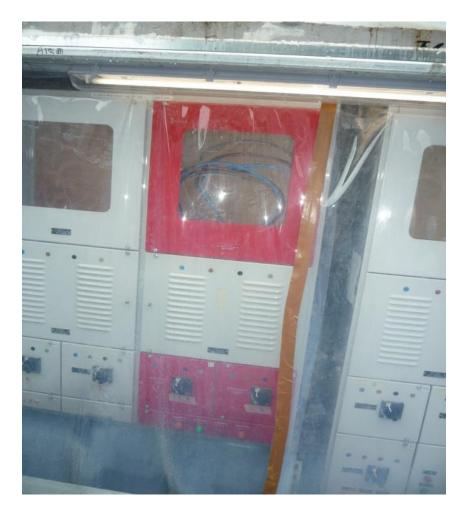
**x** Unavailable secondary power supply for FSIs and incomplete installation of supply power meter
