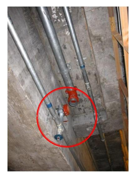
**x** Incomplete pipework of sprinkler system
