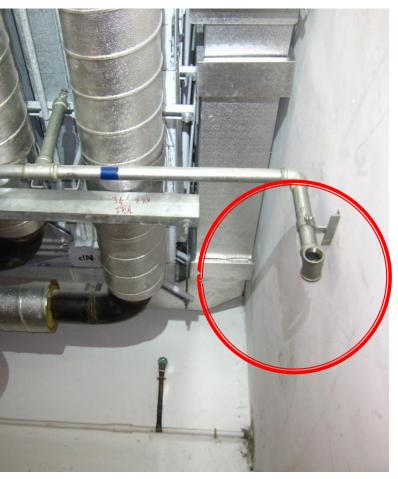
x Incomplete pipework of sprinkler system
