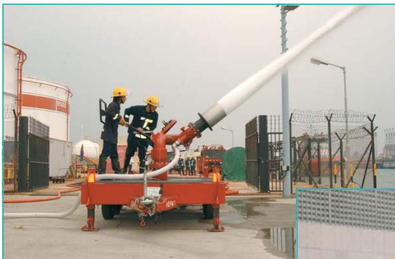
▲ 重型泡炮可應付油庫火警 Heavy duty foam monitor designed for fighting oil fires
