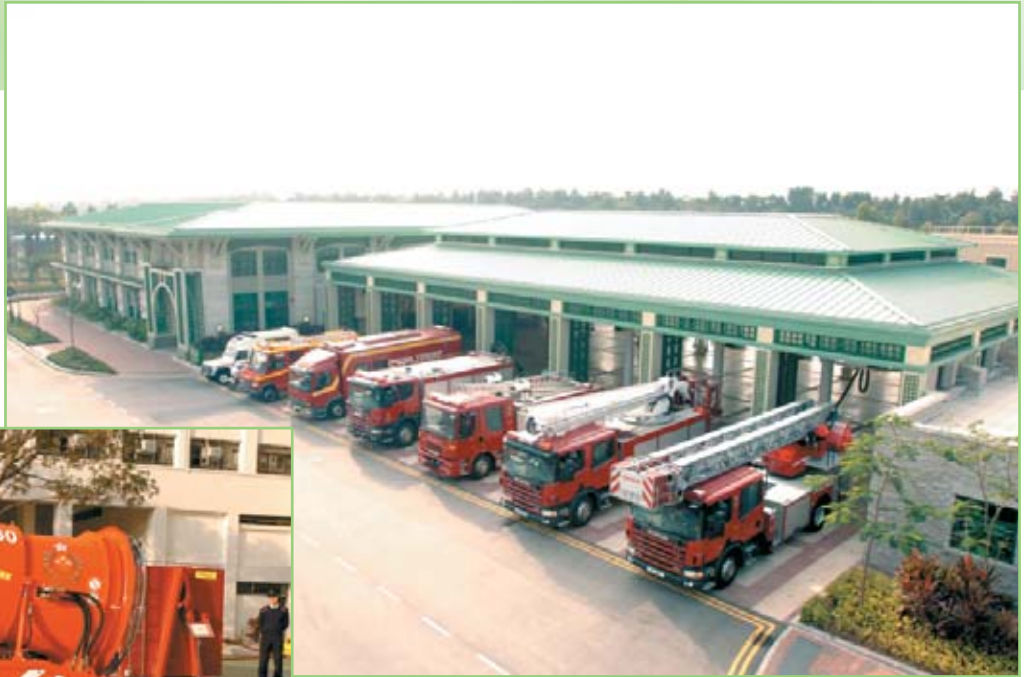
▲ 竹篙湾消防局暨救护站 Penny's Bay Fire Station cum Ambulance Depot
