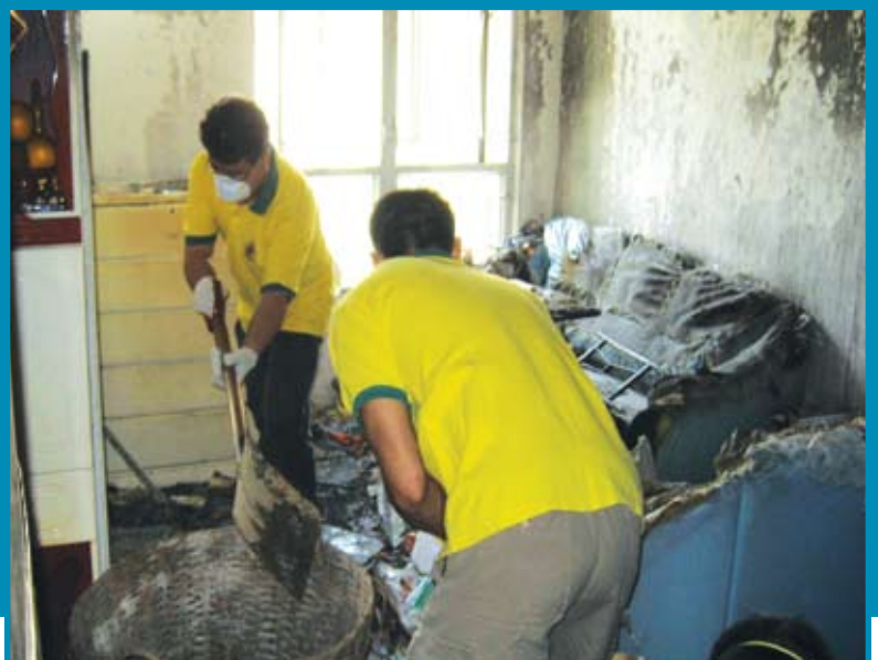
消防義工清理火災後單位 F.S. volunteers clear the unit damaged by fire
