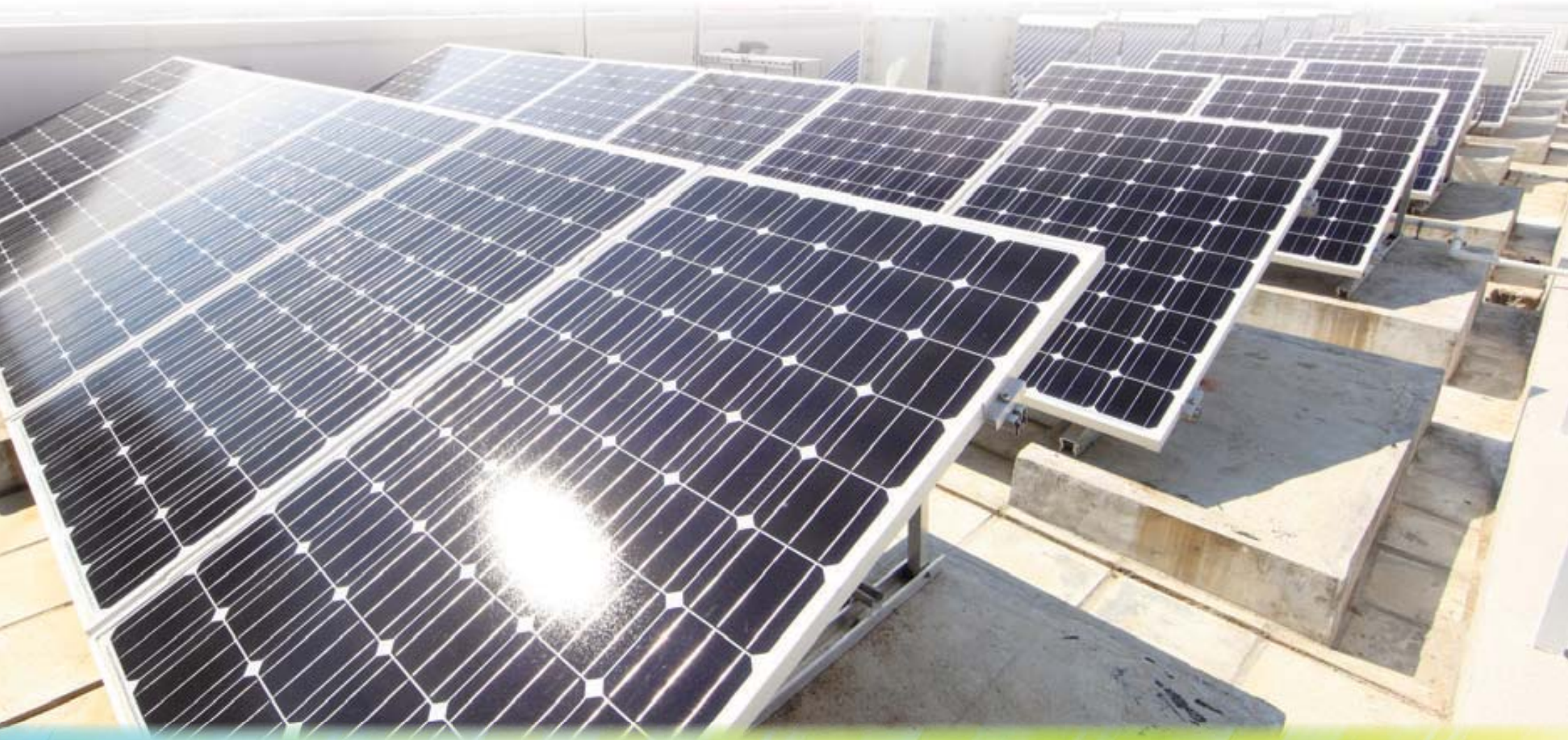
启德消防局装设光伏系统，提供环保的可再生能源 A photovoltaic system is installed in the Kai Tak Fire Station to provide renewable energy
