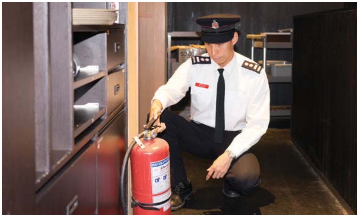
消防處人員正 檢查消防設備 A fire officer inspecting a fire service equipment
