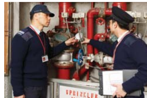
消防處人員巡查舊式樓宇的公用逃生途徑及工業樓宇的消防設備 FSD officers inspect the common means of escape of an old-style building and the fire service installations in an industrial building
