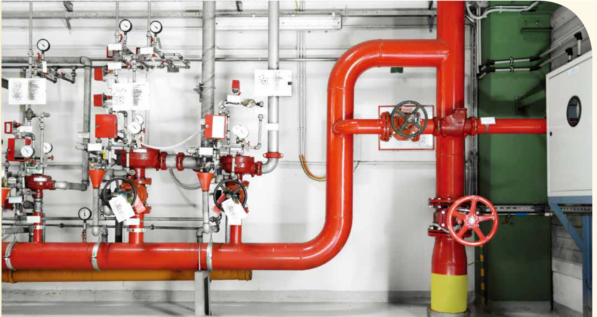
大厦的花洒系统。 A sprinkler system in a building.
