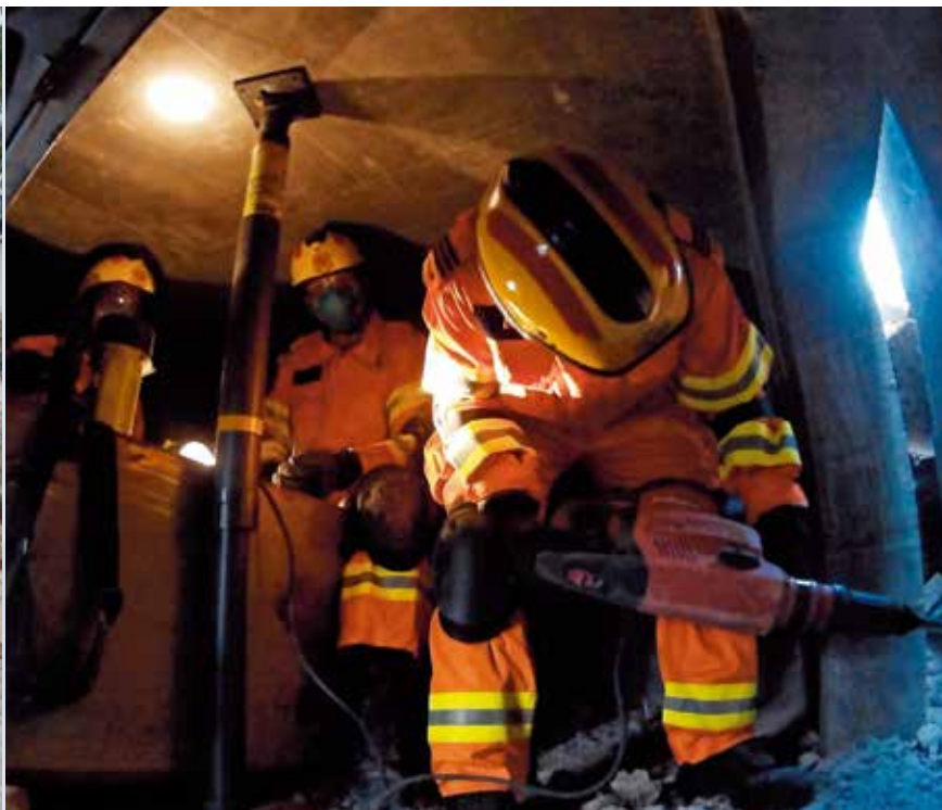
坍塌搜救專隊成員和搜救犬進行搜救訓練(左圖)；坍塌搜救專隊成員在模擬實境下進行支撐及爆破行動(右圖)。 A USAR Team member and a search dog undergoing search and rescue training (left); USAR Team members conducting a shoring and break-in operation in a simulated environment (right).
