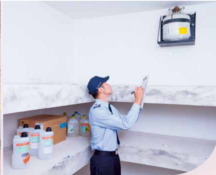
消防處人員定期巡查危險品倉庫。 Fire Services personnel inspect dangerous goods stores regularly.
