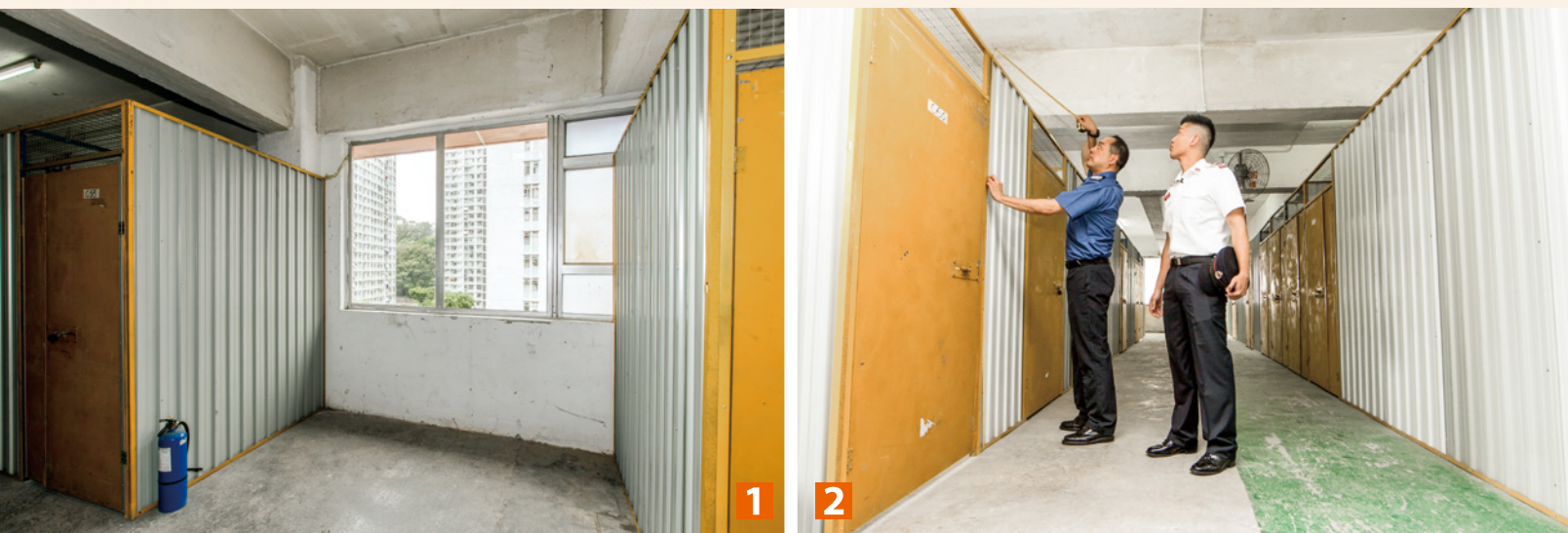
1 - 2 消防處人員到已完成改善工程的迷你倉巡查，該迷你倉的救援窗口沒有被阻塞並易於打破(圖1)，而不同貯存區域間有2.4米的分隔距離(圖2)。 FSD personnel inspect a mini-storage facility which has carried out works to comply with FSD's fire safety requirements including the provision of unobstructed and breakable access windows (photo1) and a 2.4-metre separation between mini-storage zones (photo 2).
