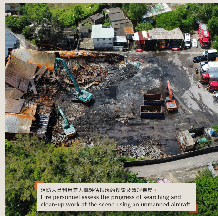
坍塌搜救專隊使用重型金屬支撐桿，穩固有倒塌危機的構築物。 The Urban Search and Rescue Team secures building structures which are in danger of collapse using heavy-duty metal props.
