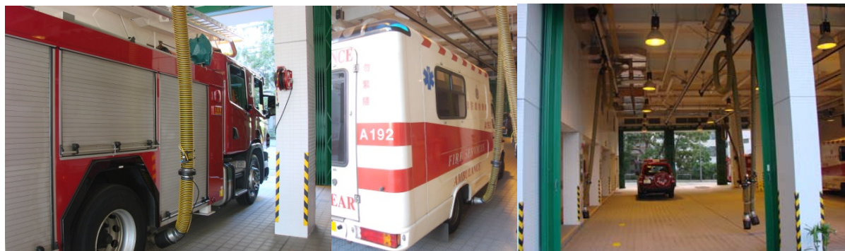
九龍塘消防局暨救護站的汽車排氣設備 Vehicle Exhaust System at Kowloon Tong Fire Station cum Ambulance Depot,
