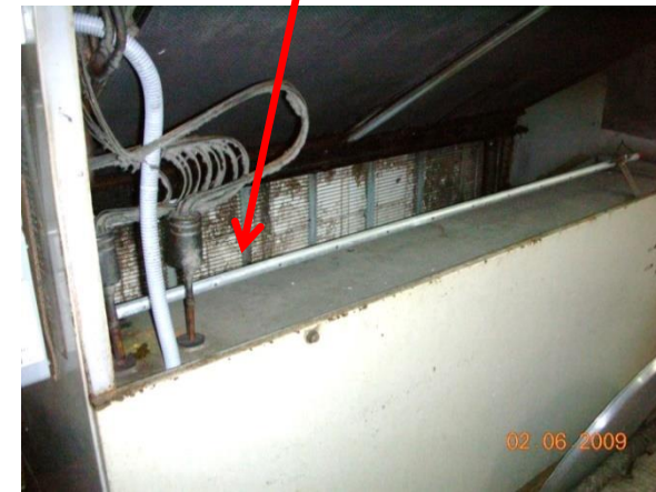
Sensing tube of probe type smoke detector
