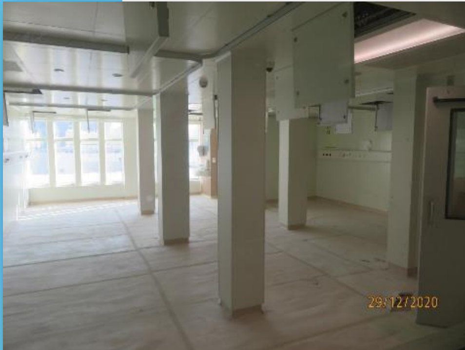
Combination of MiC units into a medical ward
