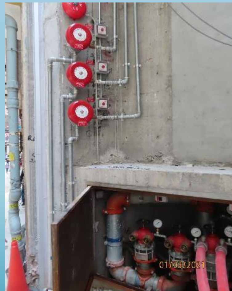
After: outside the exterior wall of the building
