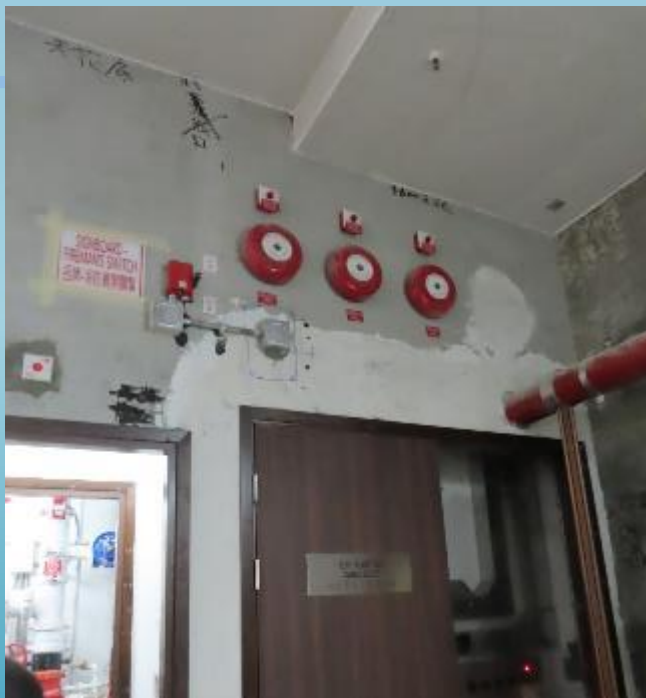
Before: inside the building
