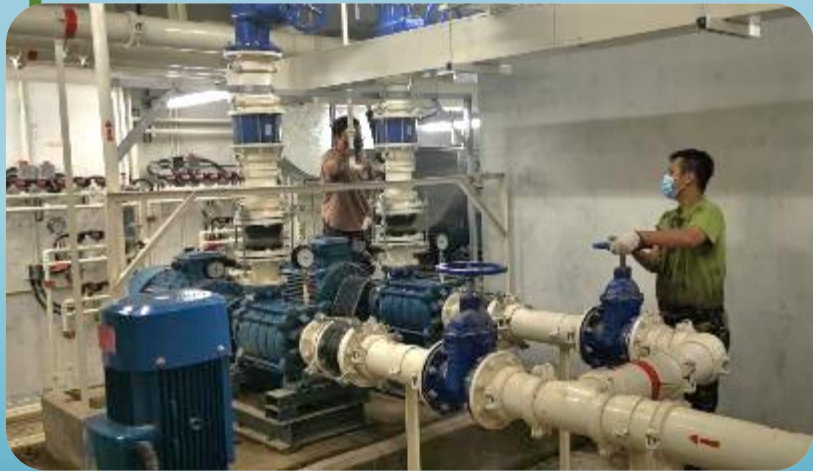
Testing and Commissioning
