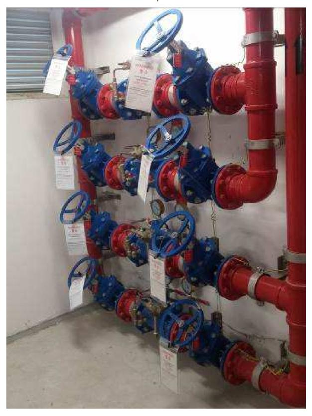
Properly-tagged SVs of an FH/HR system to avoid unauthorised operation
