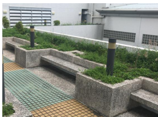
Green Roof at Kowloon Tong Fire Station
