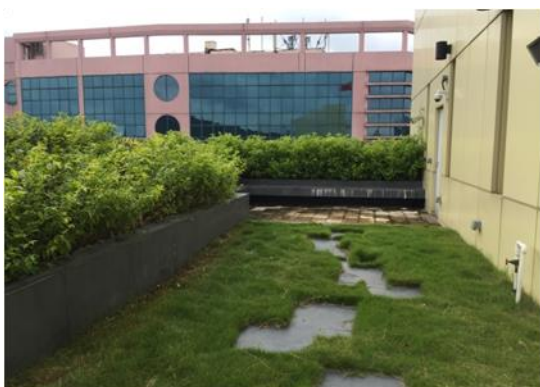
Green Roof at Sheung Shui Ambulance Depot
