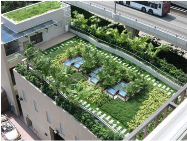
Green Roof at Kai Tak Fire Station
