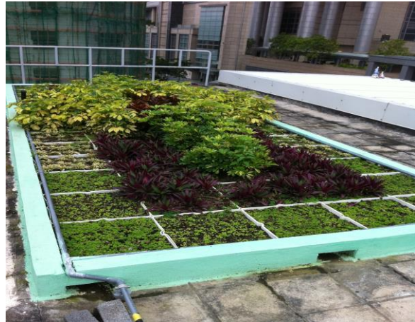
Green Roof at Kwun Tong Fire Station
