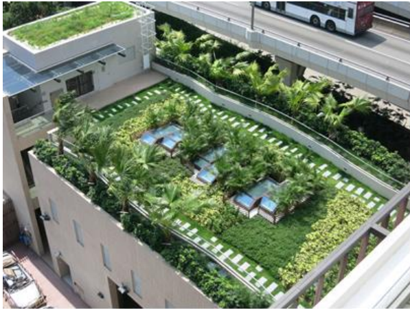
Green Roof at Kai Tak Fire Station
