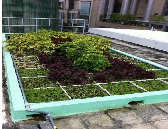
Green Roof at Kwun Tong Fire Station
