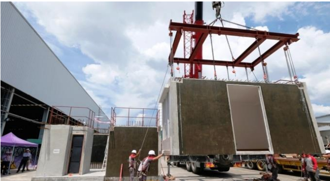
The adoption of MiC to the construction of Fire Services Department Pak Shing Kok Married Quarters
