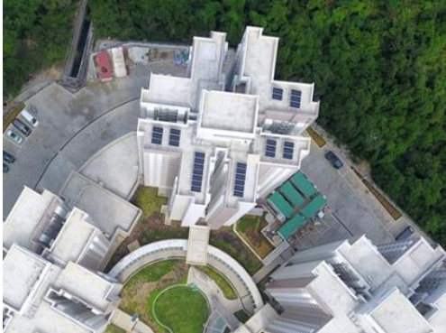
The photovoltaic panels installed in the quarters
