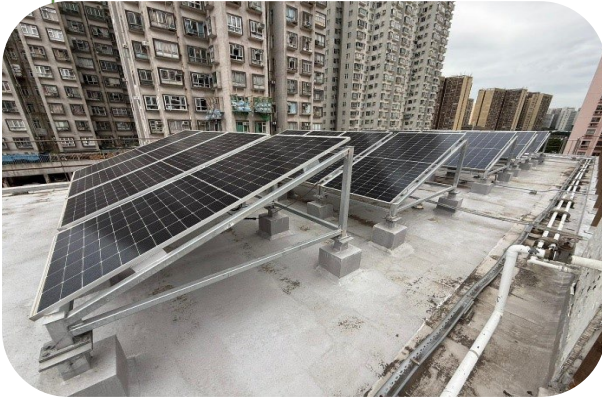
The PV panels installed at Wong Tai Sin Ambulance
