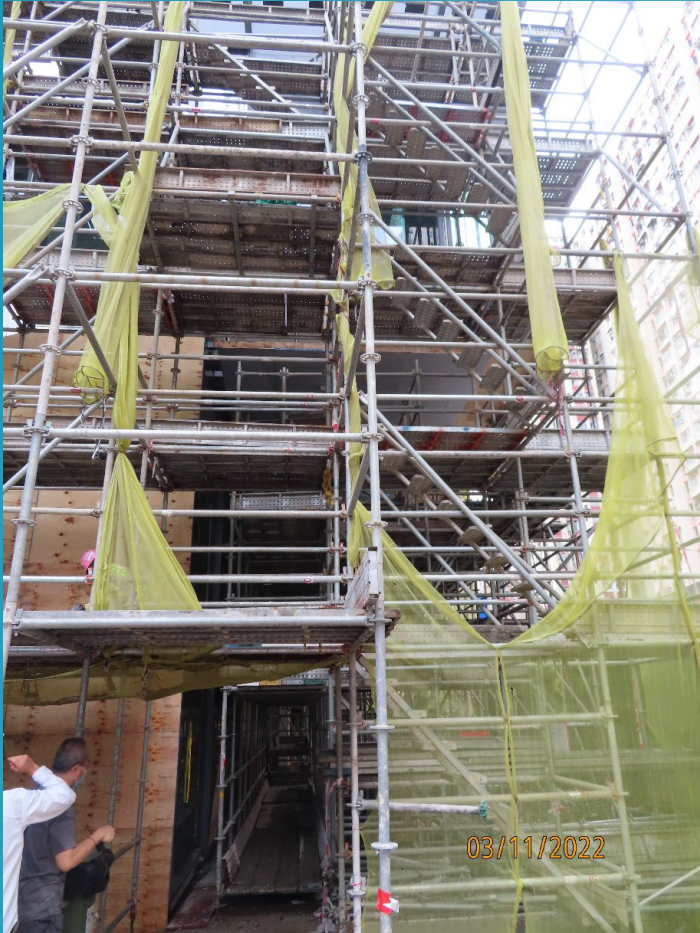
Extensive Scaffolding within inspection area
