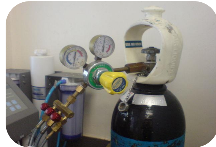
Inspected or tested by an approved person
