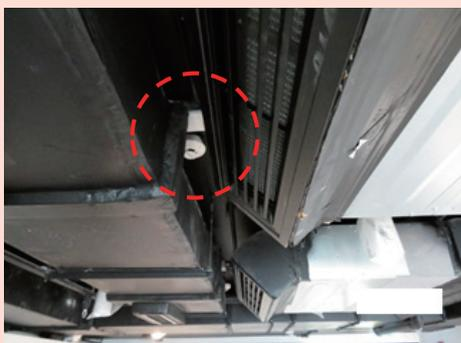
**X** Improper installation of detector (Clearance below detector should be maintained of 500 mm at least; Detectors should not be mounted within 1m of any air inlet of a forced ventilation system)
