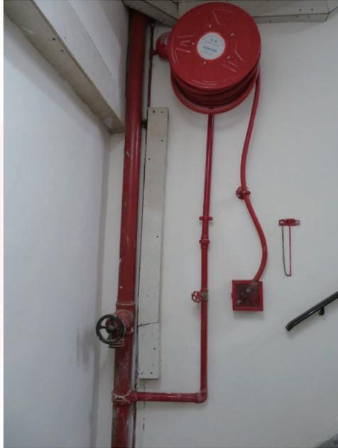
Blue label tape and notice were not stuck on the FSI that was not yet put in commission and manual fire alarm call point was not yet installed
