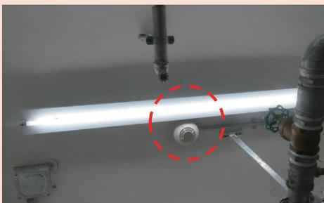
**X** Improper installation of detector (Clearance between light fitting and detector should be properly maintained in accordance with BS 5839 Part I)
