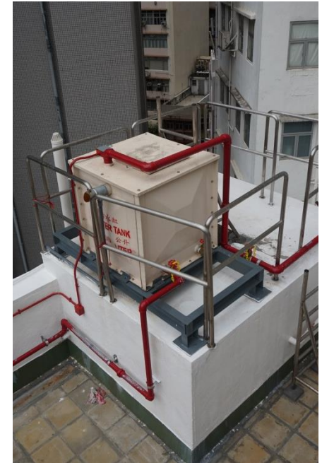
Supply Tank of 500-litre installed on Roof-floor
