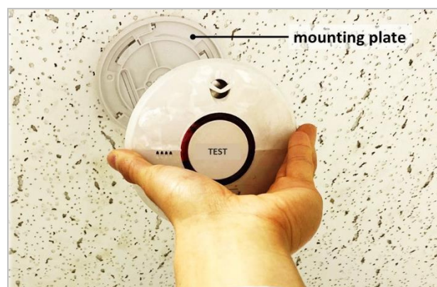
Figure 3 -A stand-alone fire detector being mounted onto mounting plate
