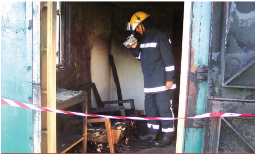
拍攝火警現場環境以進行火警調查 Fire scene video recording for fire investigation
