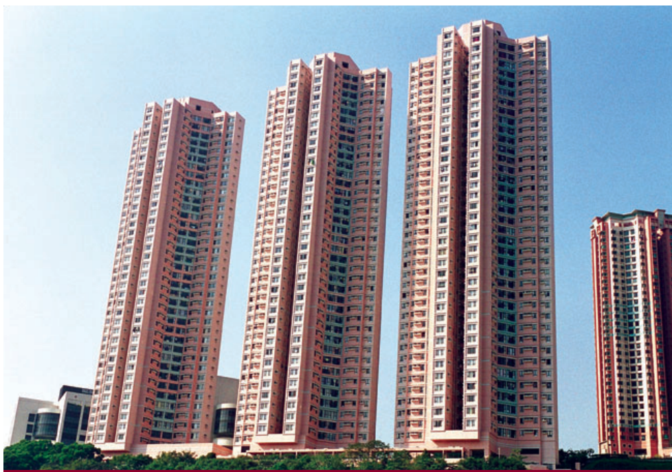
荔景纪律部队宿舍 Lai King Disciplined Services Quarters
