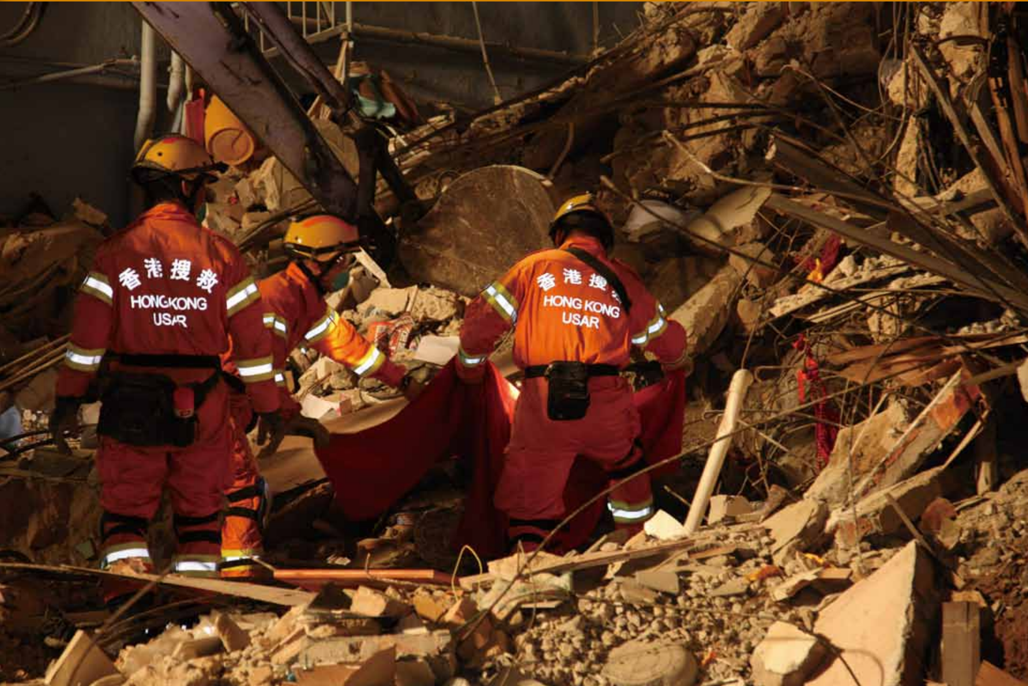
坍塌搜救专队在马头围道倒塌楼宇的瓦砾中进行搜救 The USAR Team conducts a search and rescue operation in the building collapse site at Ma Tau Wai Road
