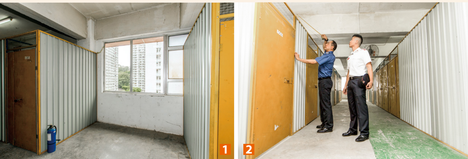
1 - 2 消防处人员到已完成改善工程的迷你仓巡查，该迷你仓的救援窗口没有被阻塞并易于打破(图1)，而不同贮存区域间有2.4米的分隔距离(图2)。 FSD personnel inspect a mini-storage facility which has carried out works to comply with FSD's fire safety requirements including the provision of unobstructed and breakable access windows (photo1) and a 2.4-metre separation between mini-storage zones (photo 2).
