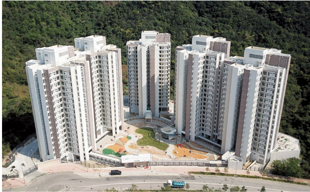
建築署圖片 Architectural Services Department photo
