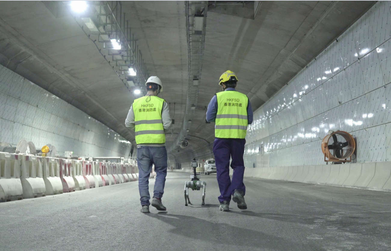
新建消防設施一站式驗收統籌辦公室的消防人員利用創新科技為中九龍繞道的消防裝置及設備進行驗收。 Fire personnel from the One-stop Coordination Office for New Fire Protection Facilities Acceptance utilise innovative technology during an acceptance inspection of fire service installations for the Central Kowloon Bypass.
