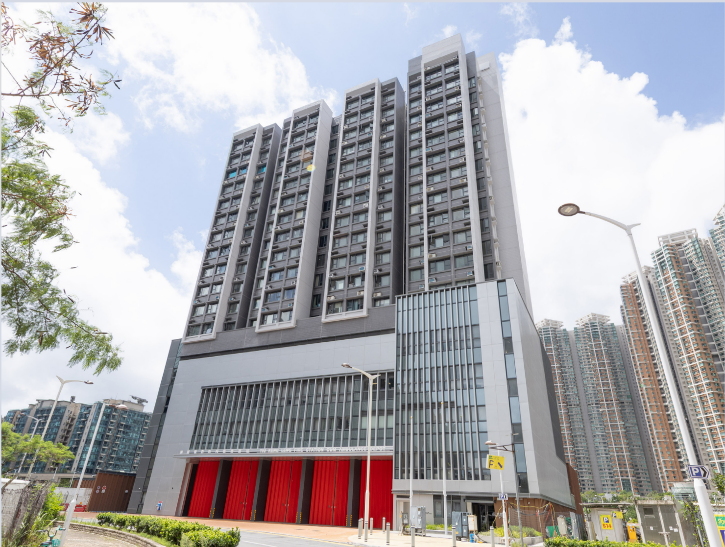
調景嶺消防局暨救護站於二零二五年十二月正式投入服務。 Tiu Keng Leng Fire Station cum Ambulance Depot has been put into commission since December 2025.
