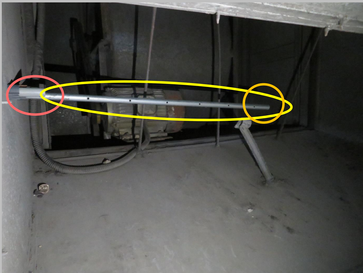
FIGURE 3. AIR DUCT DETECTOR SAMPLING TUBE:
