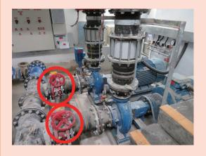
Installation of butterfly valve at the sprinkler pumps inlets
