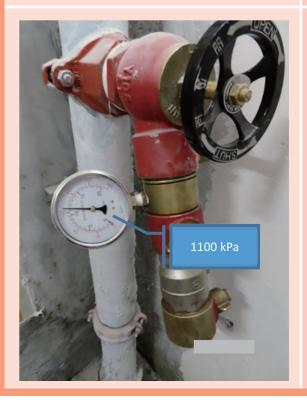
X Static pressure at hydrant outlet exceeded 850 kPa
