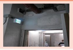
Exit sign not positioned directly above the doorway of the exit.
