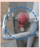
Obstruction by building structures that hamper the operation of a fire hydrant
