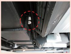
Improper installation of detector (Clearance below detector should be maintained of 500 mm at least; Detectors should not be mounted within 1m of any air inlet of a forced ventilation system)
