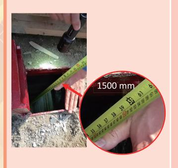
Spindle of the underground valve of a street fire hydrant more than 500 mm below valve pit cover
