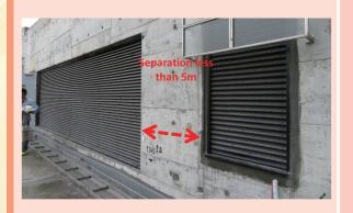
Smoke discharge (including air release of SPS) on facade less than 5000mm from other building's opening
