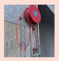
Missing of sound bell and manual call point for FH/HR System
