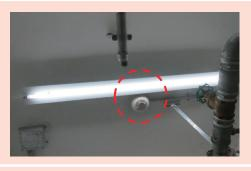
Improper installation of detector (Clearance between light fitting and detector should be properly maintained in accordance with BS 5839 Part I)
