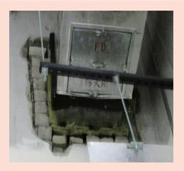
Incompletion of building works (Fire Resisting Construction)
