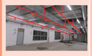
Incomplete installation of sprinkler system
