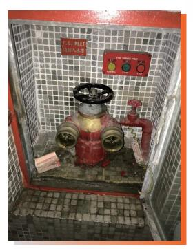
Defective Fire Service inlet noted during functional test
